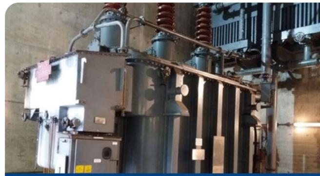
Existing internal transformers needing to be replaced (at Aigas & Kilmorack)
