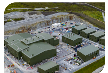
HVDC Kergord Converter Station under construction in Shetland.
