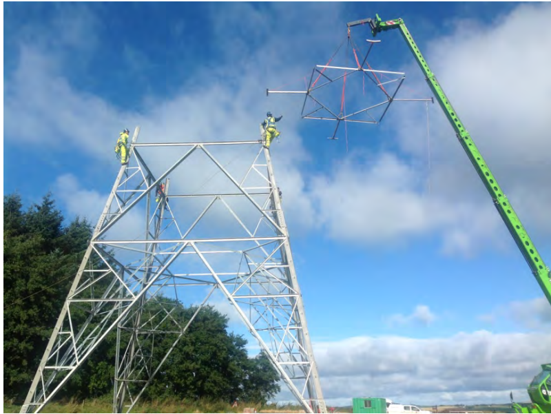
Photograph 3: Tower Assembly and Erection
