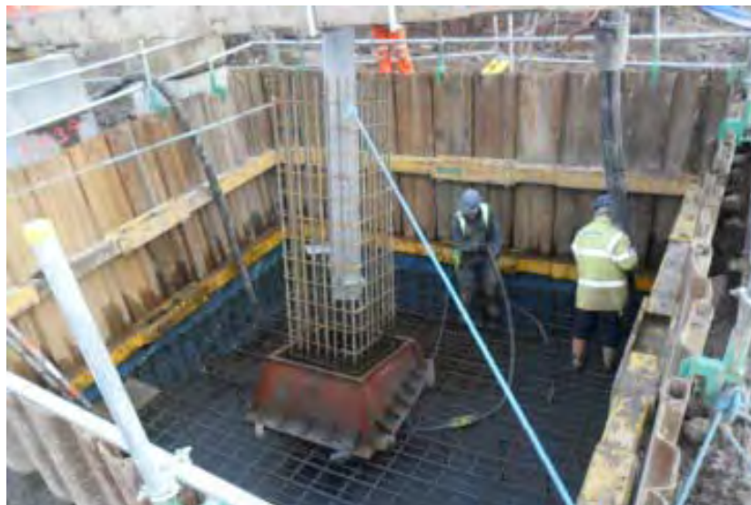
Photograph 2: Conventional Foundation Construction
