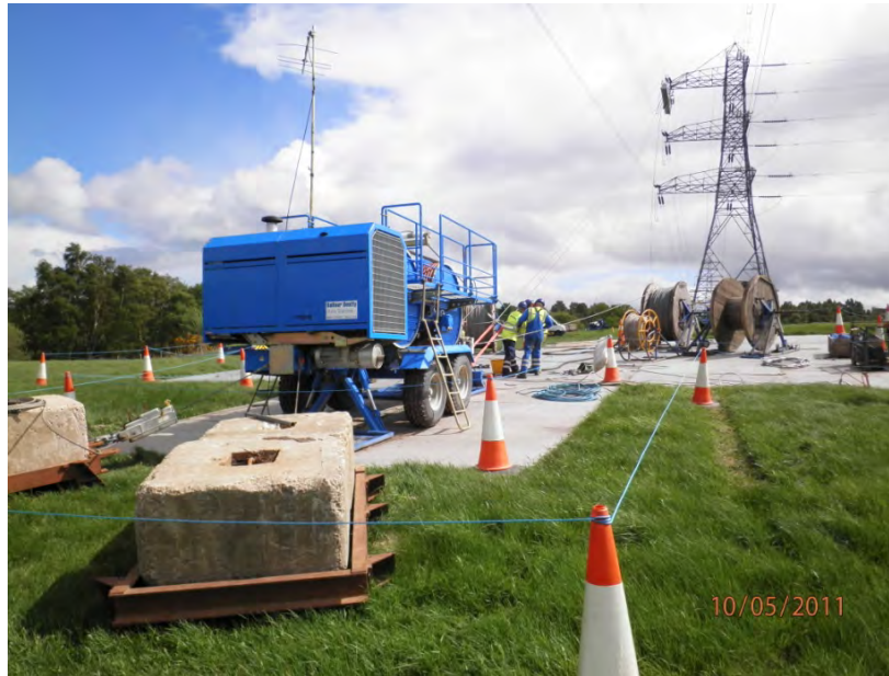
Photograph 4: Tower with Rollers and Winch, Ready for Stringing
