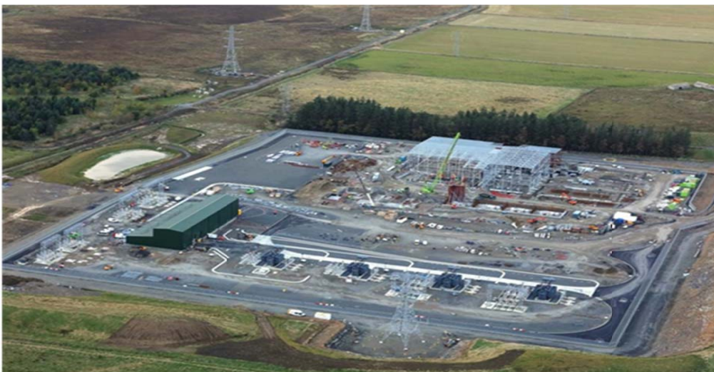
Caithness Moray – AC substation is in the foreground with converter site to the background
