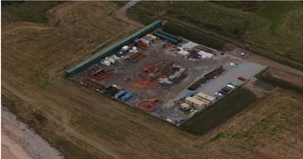
Caithness Moray – Portgordon landfall (Moray) compound during HDD operations
