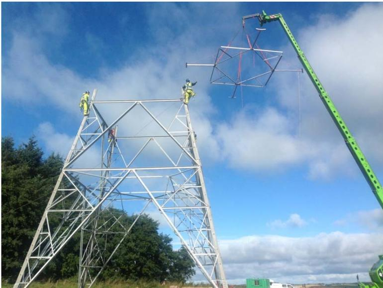
Photograph 5: Tower Assembly and Erection
