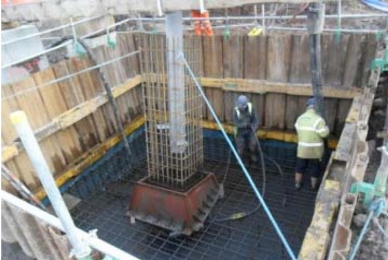
Photograph 4: Mass Gravity Foundation Construction
