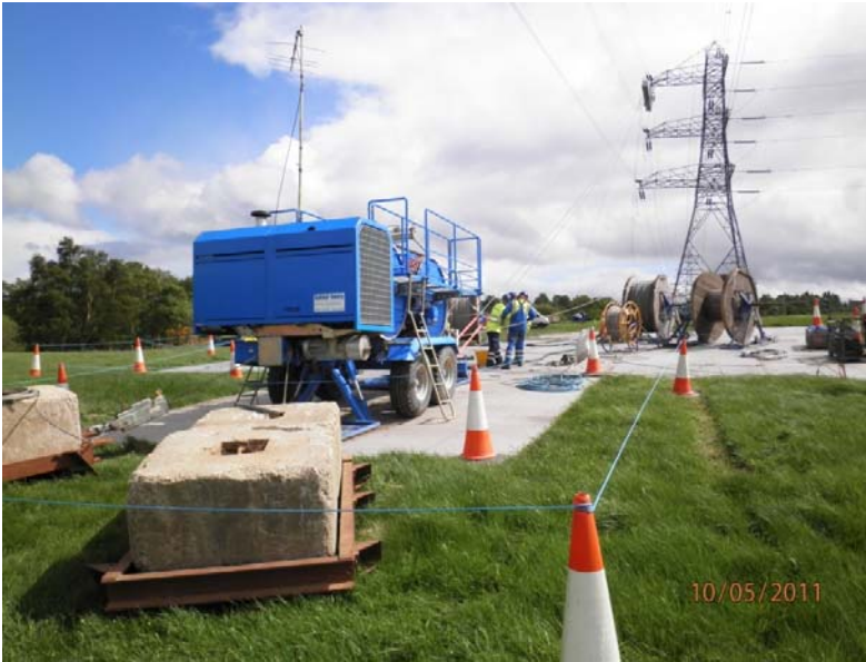
Photograph 6: Tower with Rollers and Winch, Ready for Stringing
