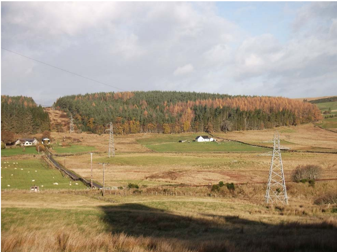
Photograph 1: Existing single circuit 132kV OHL at Gunns Plantation
