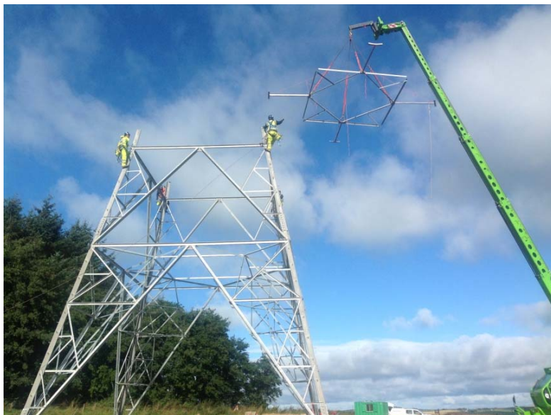
Photograph 5: Tower Assembly and Erection
