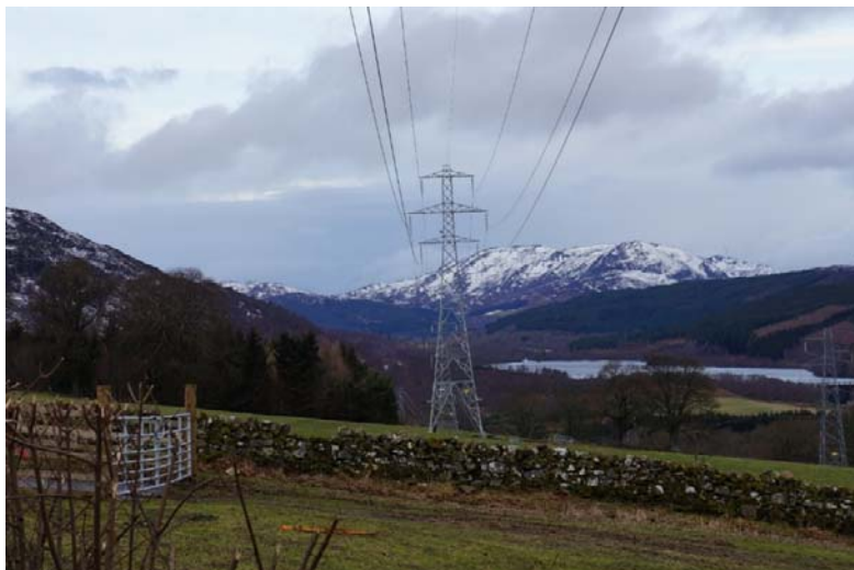
Photograph 2: Typical new build 132kV OHL.
