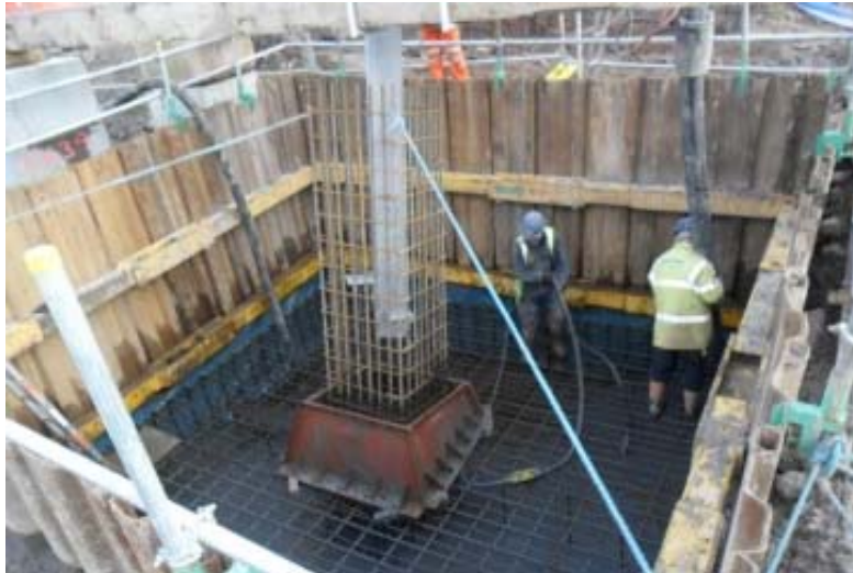
Photograph 4: Mass Gravity Foundation Construction
