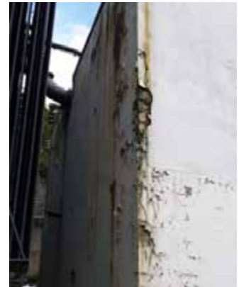
Fire wall degradation, St Fillans PS
