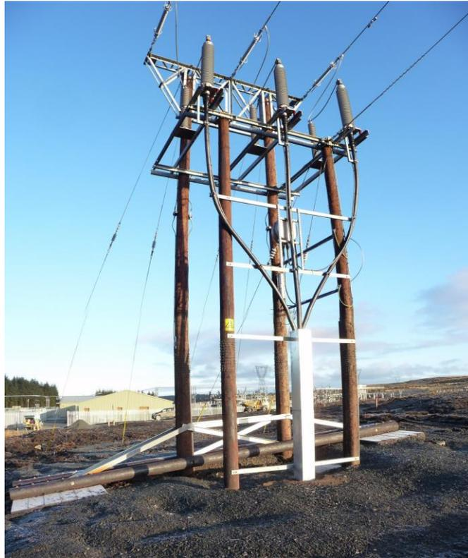
**Photograph 3.2: Typical Sealing End Structure**
