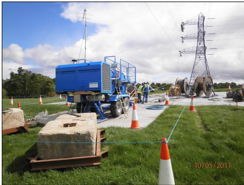
**Photograph 2.1 Typical EPZ with equipment set up for re-conductoring**
