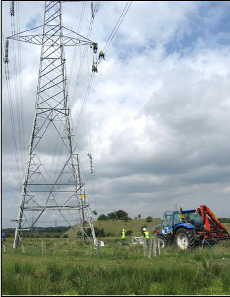
**Photograph 2.2: Replacing insulators on an existing OHL tower**
