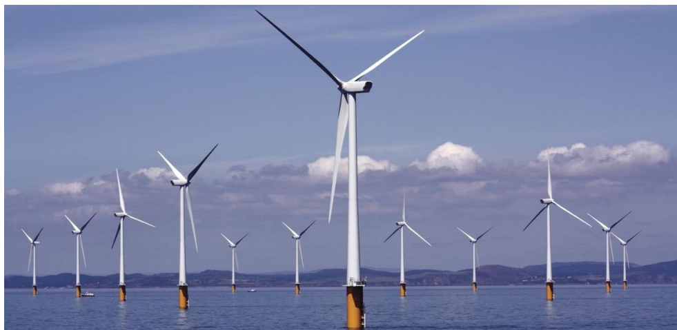
1 One of the increasing numbers of offshore wind farms being built as we move to a renewable based power system.
